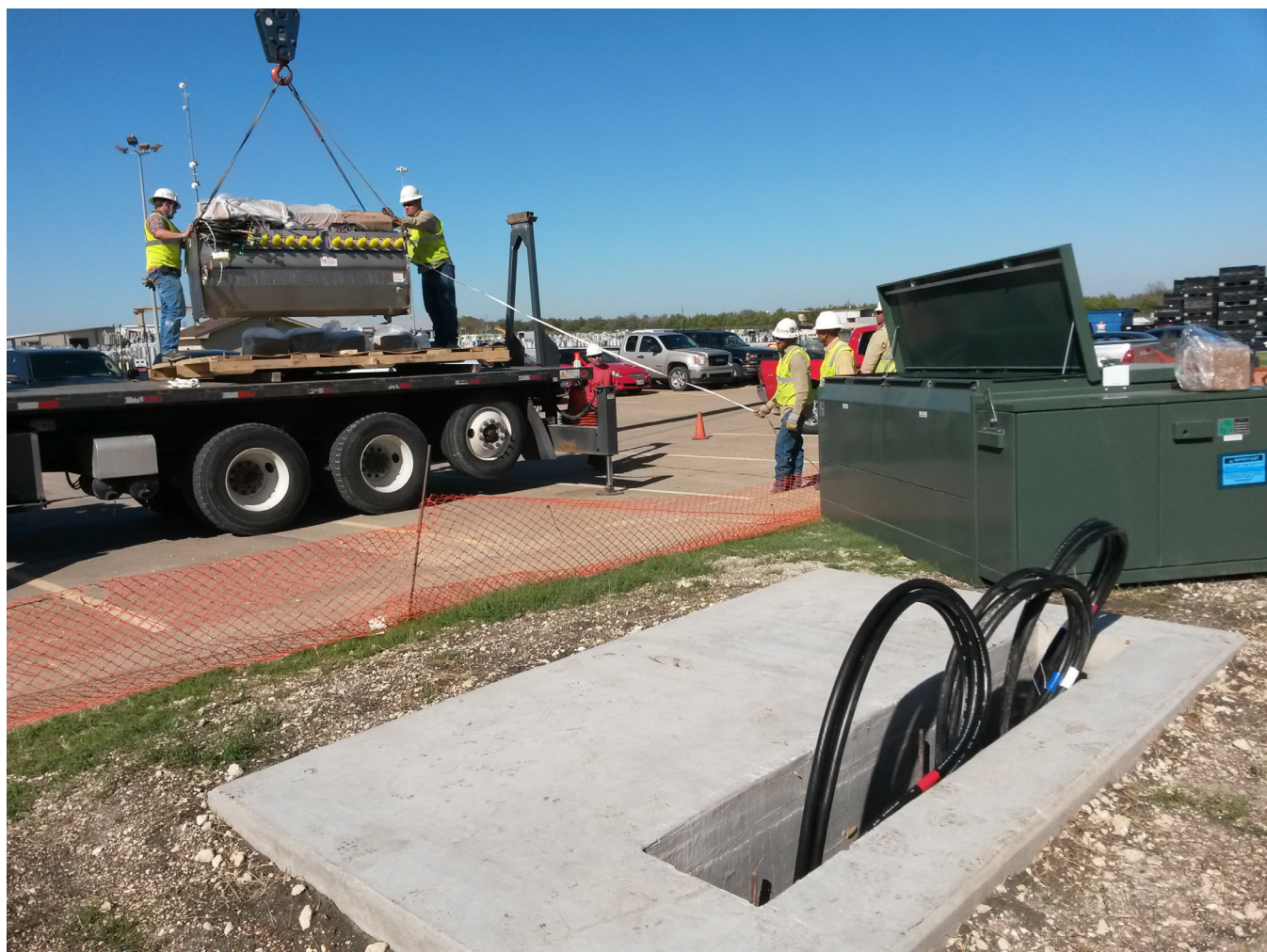
Crews install S&C Vista® Underground Distribution Switchgear.
